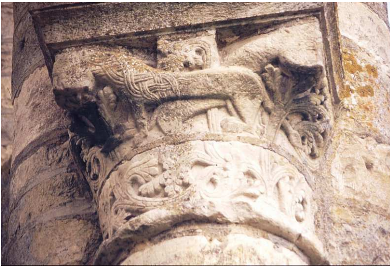
Charroux (86) - Capital on remains of rotunda
